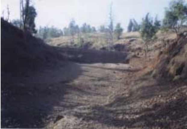
Small lake & Checkdam at Ozarda - Batada village made during Jan-Feb., 2002.
